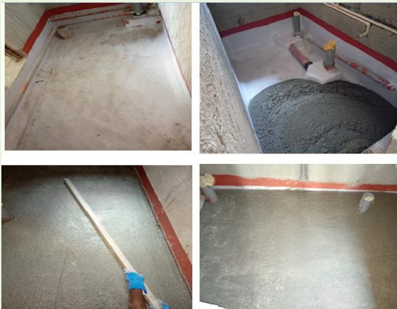
Project site execution of Elitecrete™
