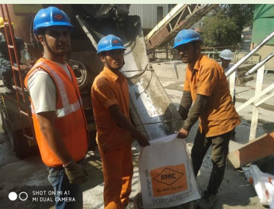
Filling up of Portacrete® bags
