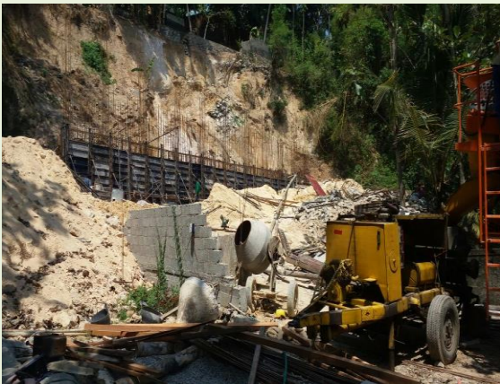
Easycrete® execution site
