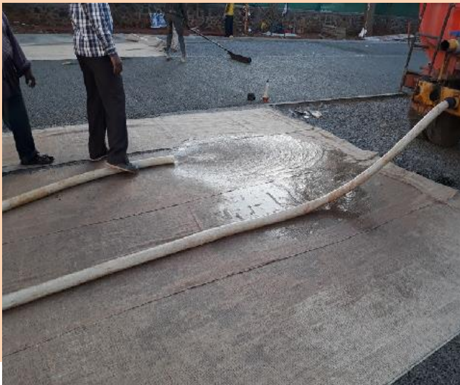
CURING BY JUTE SHEETS
