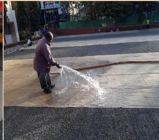
CURING BY JUTE SHEETS
