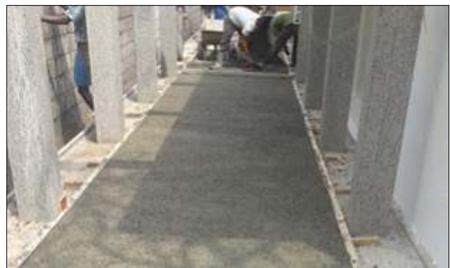
Fig. 4 Laying of Perviouscrete ™
