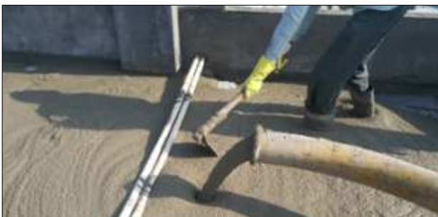
Fig. 2 Elitecrete ™ being pumped on the roof slab
