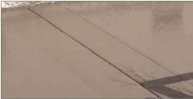
Fig. 1 Typical close-up of a joint
