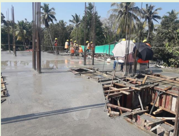
FRCcrete® execution on slab
