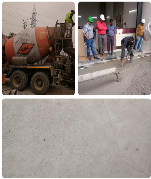
Elitecrete™ as a filler material at ground floor
