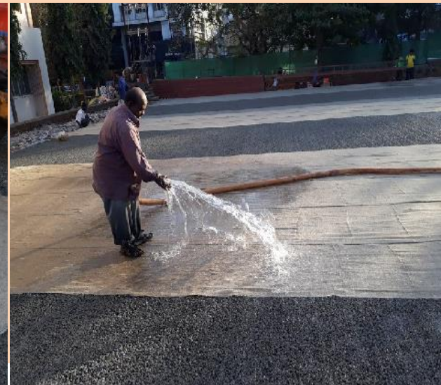
CURING BY JUTE SHEETS
