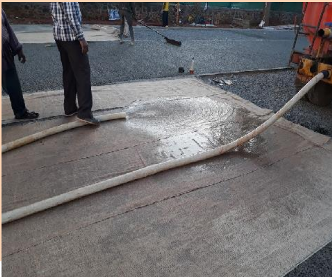
CURING BY JUTE SHEETS
