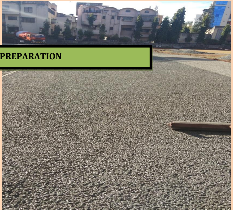
PLACING OF PERCIUSCRETE™
