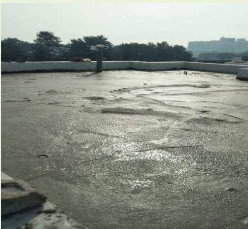
Execution of Elitecrete™
