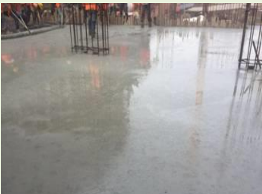
Photographs of Beam and finish Slab.
