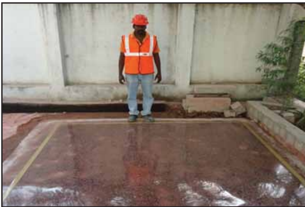
Fig 2 Polished concrete panel at Chennai
