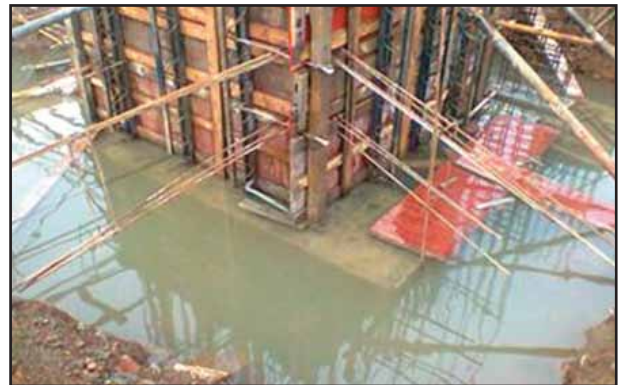
Fig 4: Anti wash-out concrete had set properly within 24 hours and work on further lifts could start immediately
