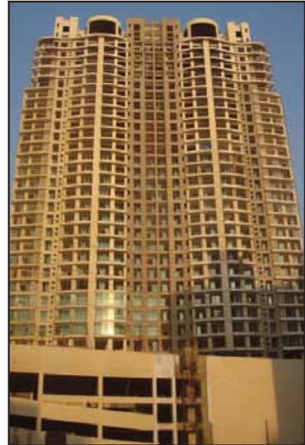
Fig 3 Windsor, Jogeshwari: Concrete was pumped up to 35 th storey
