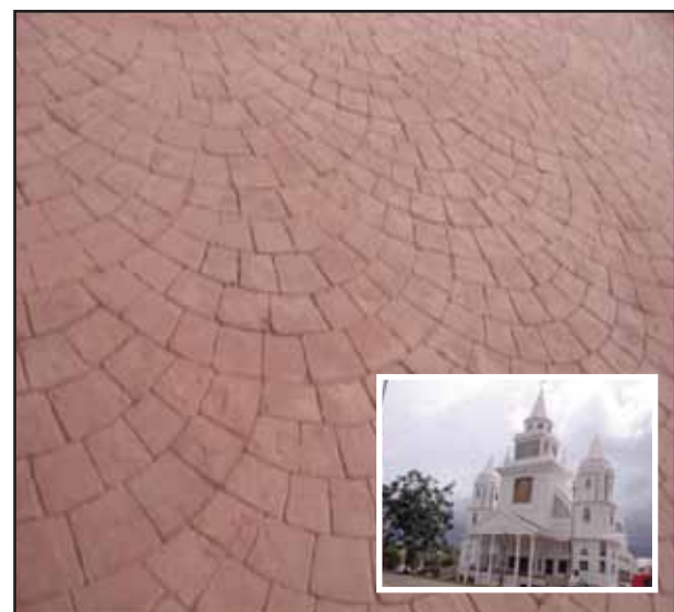
Fig 1 Stamped concrete application at Kochi (Inset-Rajagiri Church)
