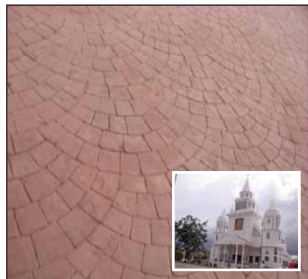
Fig 1 Stamped concrete application at Kochi (Inset-Rajagiri Church)
