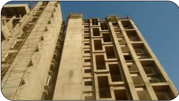
Typical high-rise building constructed with *Readyspread*<sup>®</sup> and Mivan formwork
