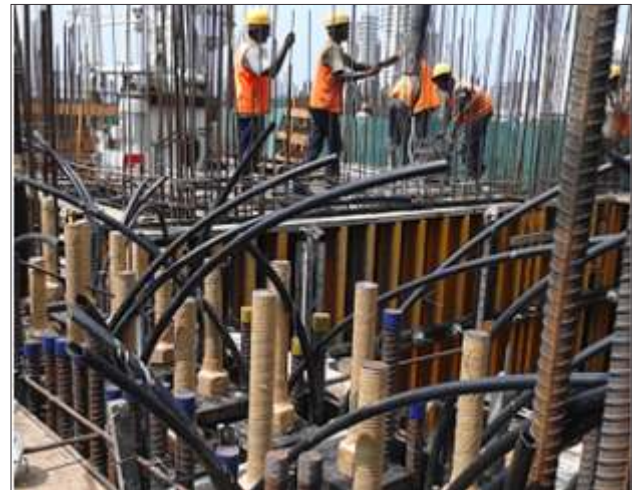
Fig. 1 Megacrete® being placed in forms
