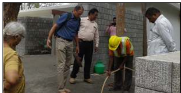
Fig. 5 Testing of Perviouscrete ™
