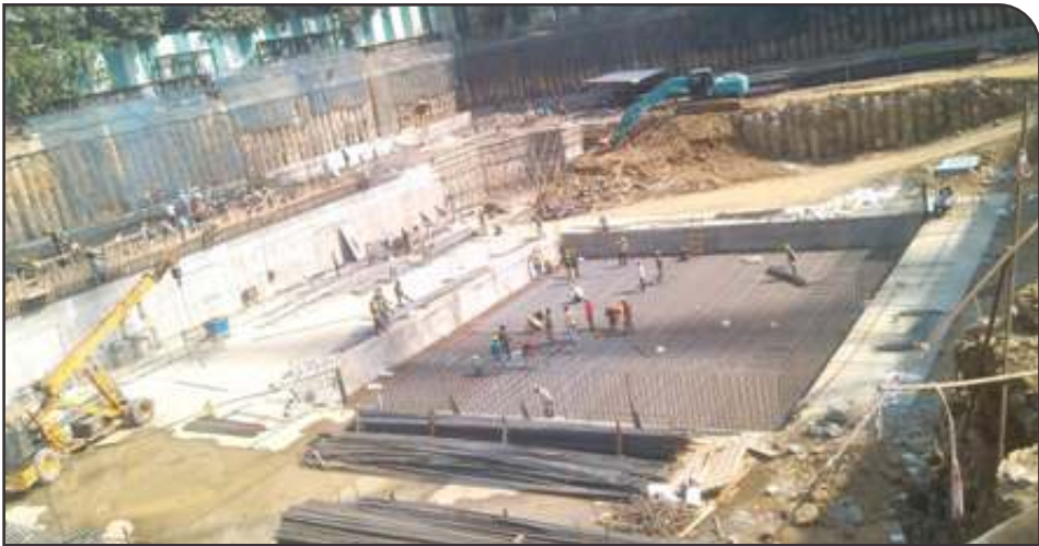
Fig 2 Easycrrete™ being pumped in the raft foundations
