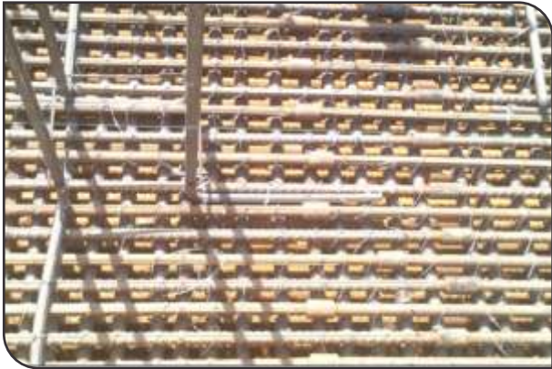
Fig 1 Close up of congested reinforcement in the raft foundation
