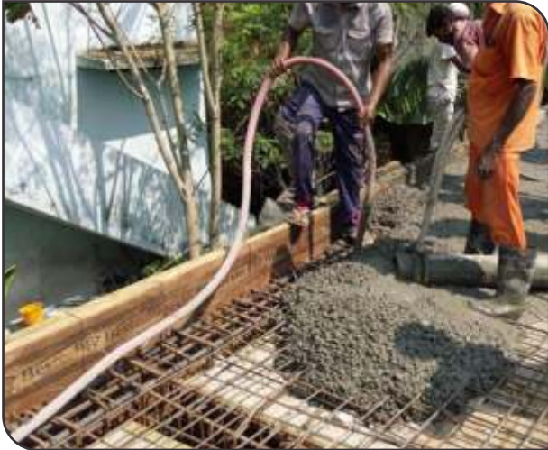
Concrete with copper slag as partially replaced fine aggregates
