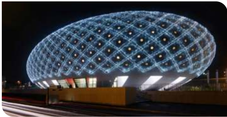
Centro Ovale concrete shell, Chiasso, Switzerland, illustrates the versatility of concrete'
