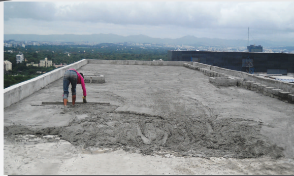
Elitecrete™ being laid on a terrace slab.
