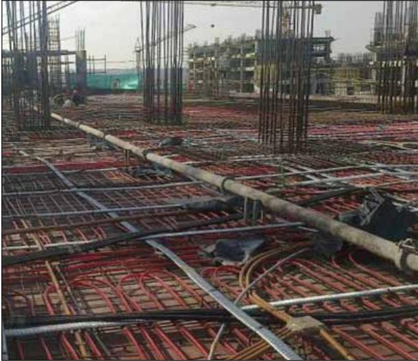
*Fig 2 Network of Pipes (red colour) tied to reinforcement and placed in position before concreting of slab*
