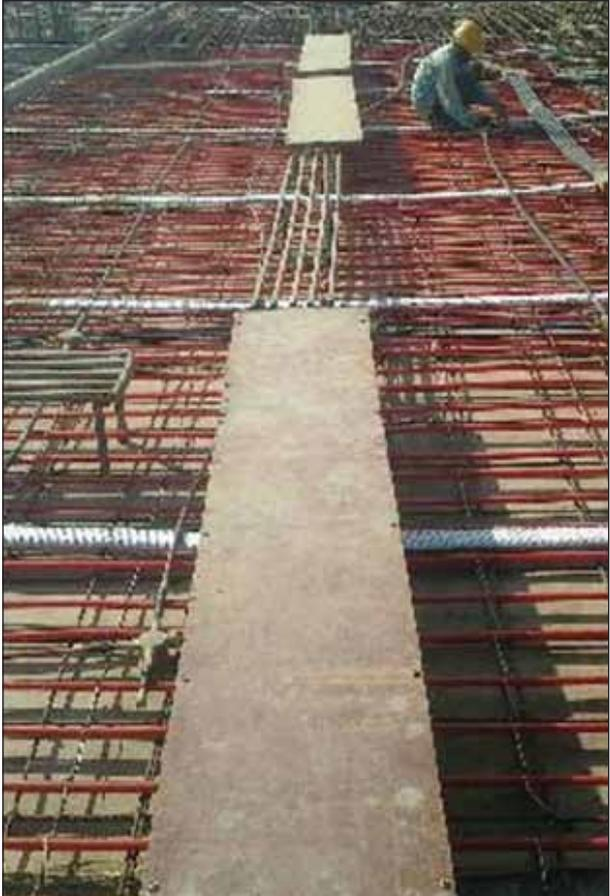
*Fig 4 Platform laid on strands to carry workmen and pumping pipes*
